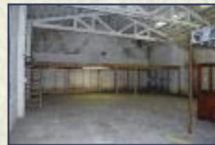
Raw adjoining space. To be used for expansion in the future. Good for larger events and/or rental space.
